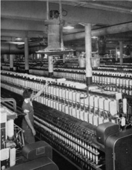
Figure 2. A Ring-Spinning Frame, c. 1940
