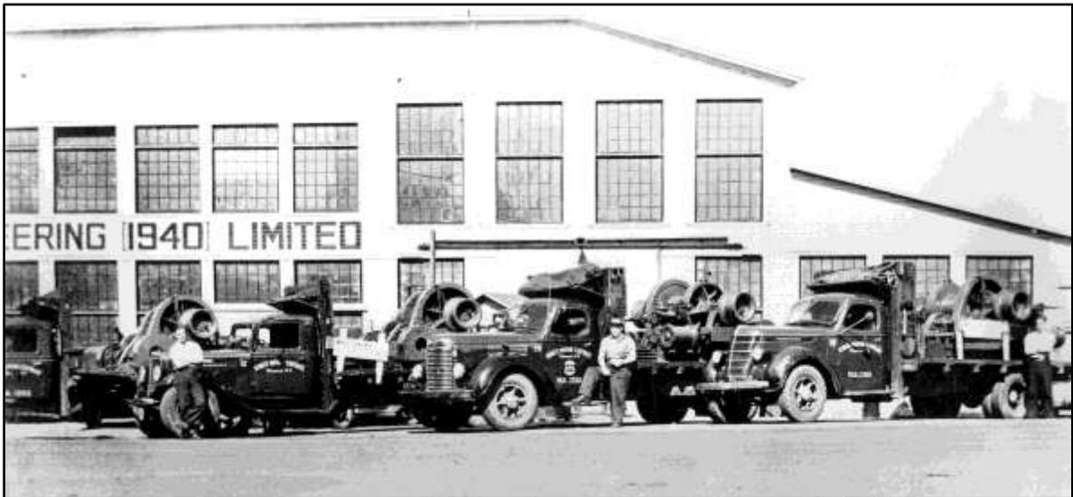
Windlasses manufactured by Heaps Engineering (1940) Limited loaded onto flatbed trucks for delivery to nearby Vancouver shipyards to meet progress schedules. Wartime saw more extensive use of subcontracting to industrial firms and pre-fabrication of components in British Columbia's Lower Mainland. (New Westminster Public Library)
