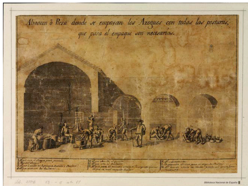
Figure 1: Packing warehouses for quicksilver in Almadén, Spain.
